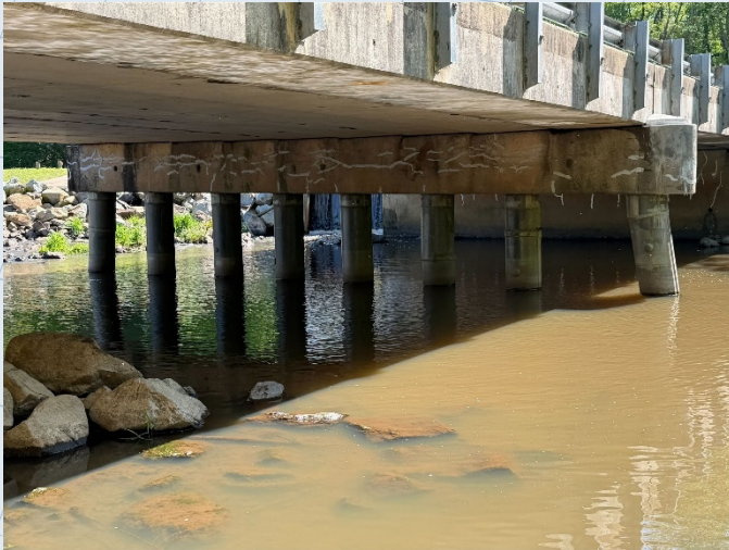
View of full bent after repairs and fiber-reinforced polymer jacket placement on a recently repaired bridge
