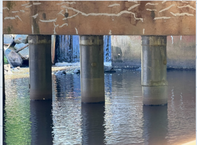
Close up view of fiber-reinforced polymer jackets on a recently repaired bridge
