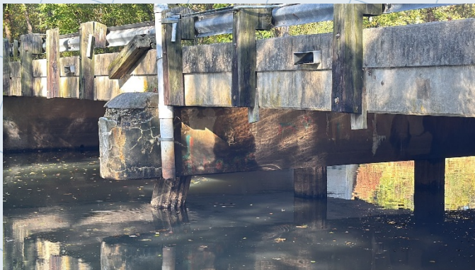
View of the South Bent Cap and the West Abutment
