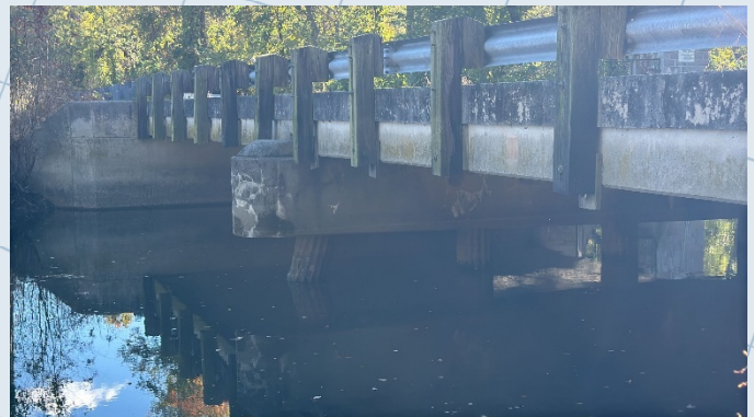
View of the North Bent Cap and the East Abutment
